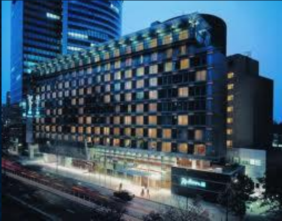
Radisson Blu Centrum Hotel (311 rooms)
