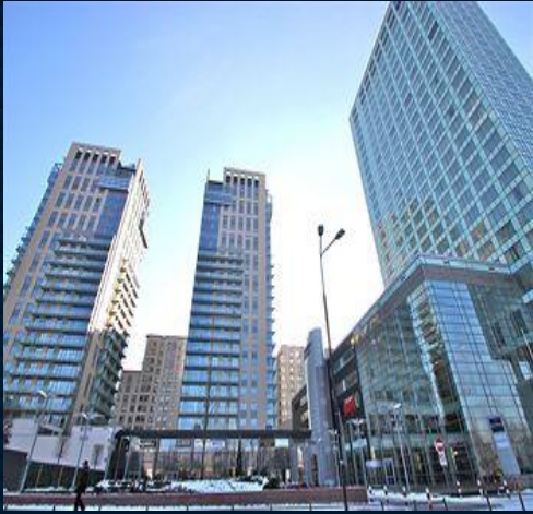
Platinum Residence (217 rooms)
